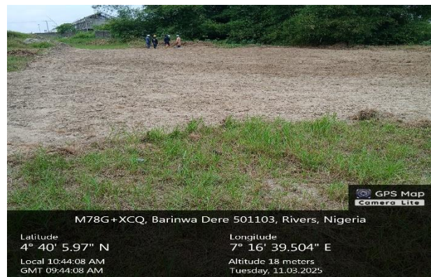
Excavated and tilled area
